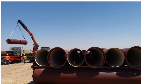
Ductile Iron Pipes Accessed to Gaza and Installed on Site for UNDP Package in June and July 2018
