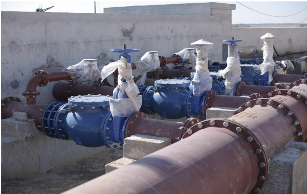
Installed High Density Polyethylene Pipes and Valves for Drying Beds up to December 2018
