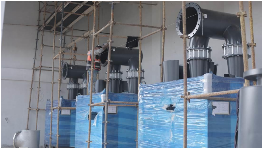
Installation of Air Blowers in the Air Blowers Room in December 2018
