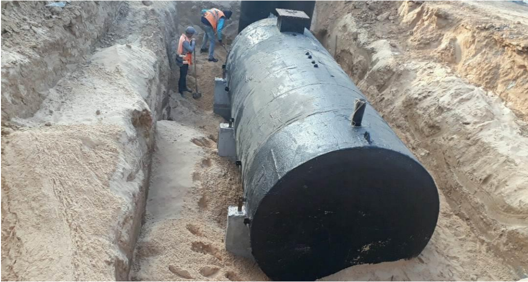
Installation of Fuel Tank for KY WWTP in December 2018
