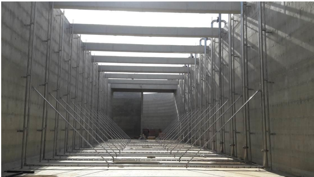
Mechanical Installation for the Aeration Tank in December 2018
