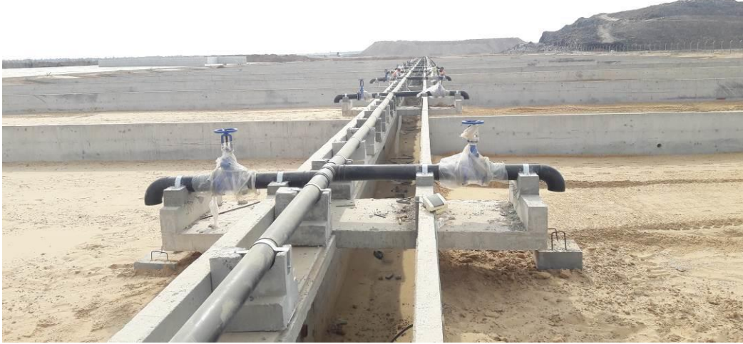
Installed High Density Polyethylene Pipes and Valves for Drying Beds up to December 2018
