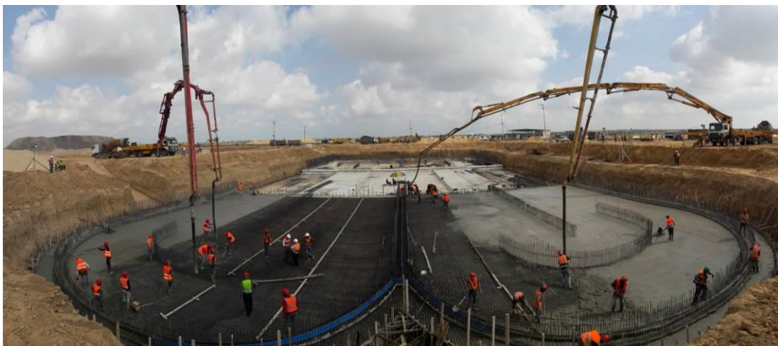
Casting Reinforced Concrete for the Foundation of the Aeration Tank on 20 June 2017
