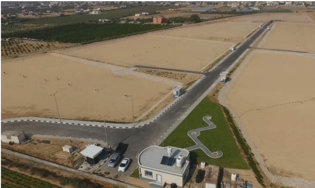
Accomplished Works of the Infiltration Basins up to November 2018
