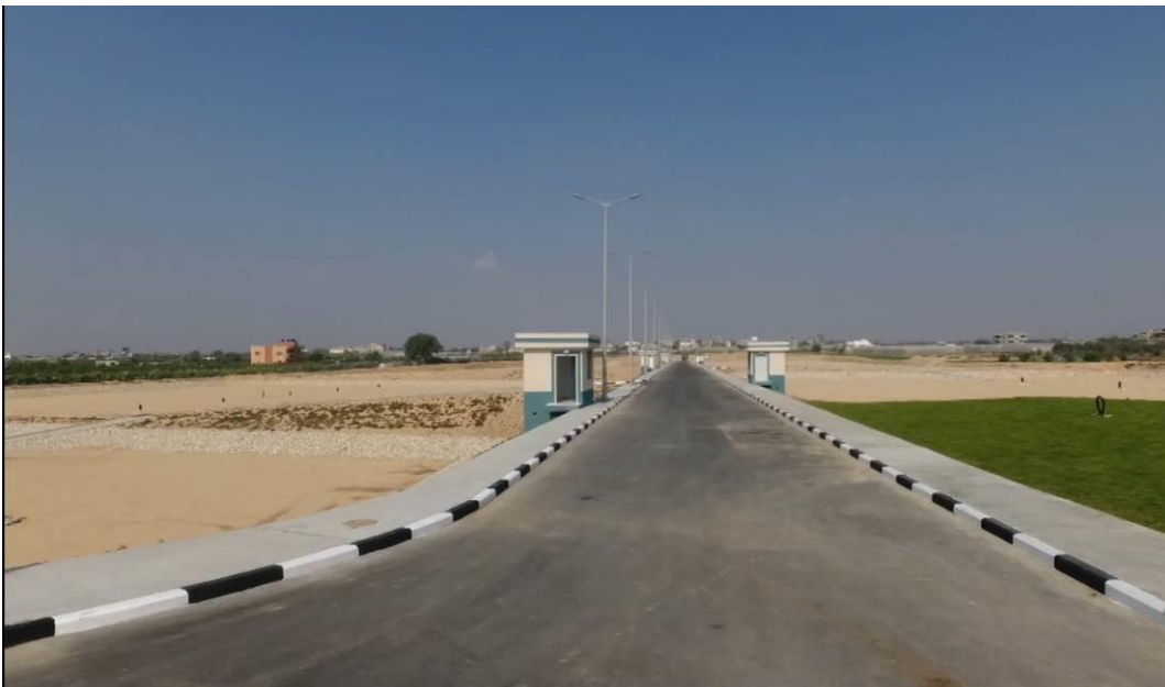
Accomplished Works of the Infiltration Basins up to November 2018
