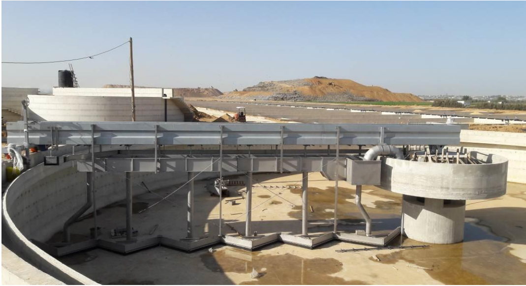
Mechanical Installations for the Clarifiers in December 2018
