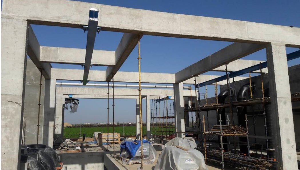
Mechanical Installations for the Sand Filter in December 2018
