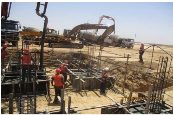
Starting Casting Reinforced Concrete for Admin Building and Plain Concrete for Aeration Tank on 17 May 2017
