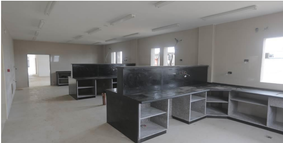
Finishing Works for the Lab in the Administrative Building in December 2018
