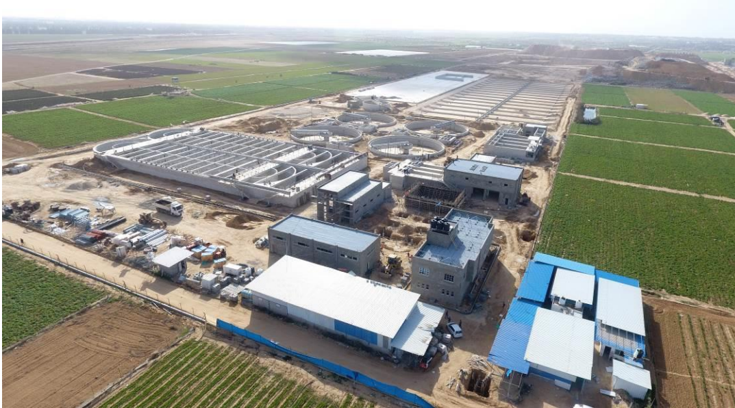
General View for Accomplished Works of KY WWTP in December 2018
