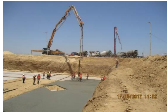
Starting Casting Reinforced Concrete for Admin Building and Plain Concrete for Aeration Tank on 17 May 2017
